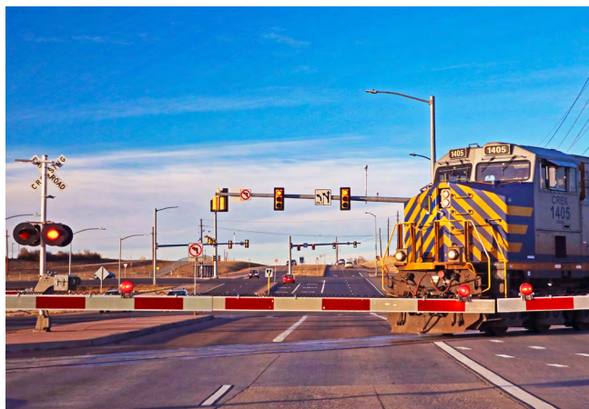
Figure 31. Active Railroad Warning Devices
