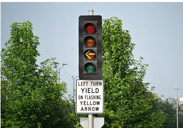
Figure 18. Flashing Arrow Signal
