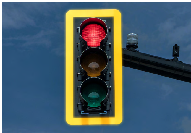
Figure 8. Retroreflective Backplates
