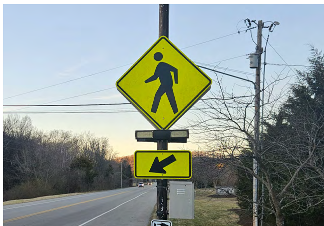
Figure 21. Rectangular Rapid Flashing Beacon (RRFB)
