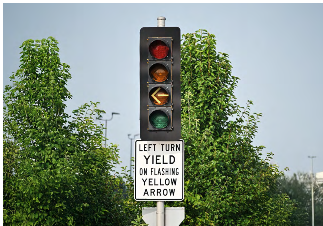
Figure 18. Flashing Arrow Signal
